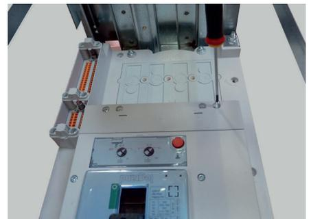
Fix them using the screws supplied (two per terminal shield).
