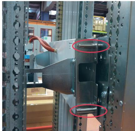
The 4 guide pins make it easier to position the movable part on the fixed part, as it ensures that the connector pins are perfectly adjusted.
