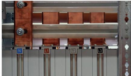
Don't forget to fix the busbar identification plate at the top of the chassis.
