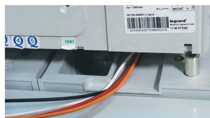
When installing the circuit breaker, space is left on the base to allow the wires to exit.
