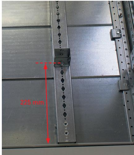
Screw the upright fixing lugs to the top and bottom crosspieces (225 mm from the front of the enclosure).
