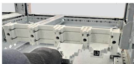
The bottom support takes the busbar end stops, which slide into a groove in the insulator.
