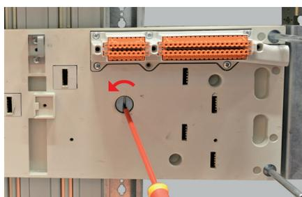
The fixed part is locked with 1/4 turn screws.
