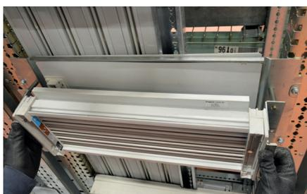
Insert the movable part in the fixed part with the aid of the guide pins.
