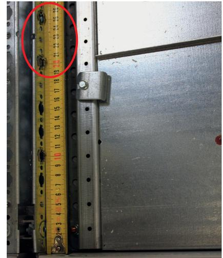
To secure the functional uprights, insert the clip-nuts 200 and 250 mm from the front.
