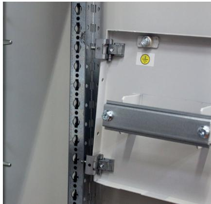
After screwing both hinges onto the faceplate as indicated in the instructions, the assembly is fixed on the faceplate support upright using both nuts supplied.
