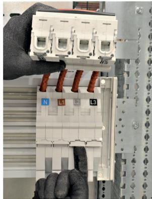
While holding the circuit breaker with one hand, install the base on the HX<sup>3</sup> IS 400 A row distribution block and activate the locking levers.
