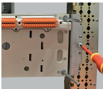
The fixed part of the base is finally secured on the VX<sup>3</sup> IS chassis uprights using the two screws supplied (don't forget to insert the two clip-nuts in the uprights first).
