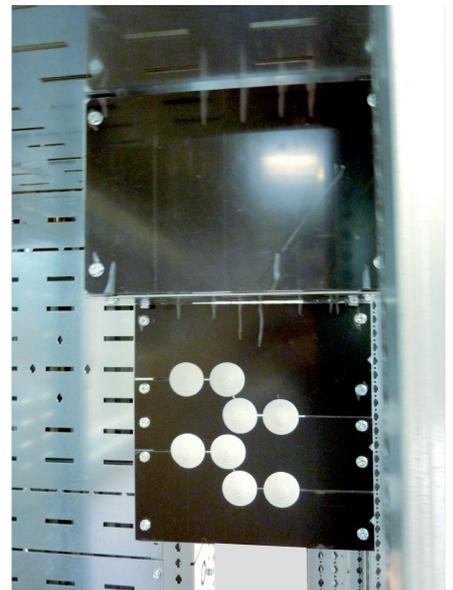
Equipped in this way, the IS system ensures compliance with the requirements of 4b form of separation.
