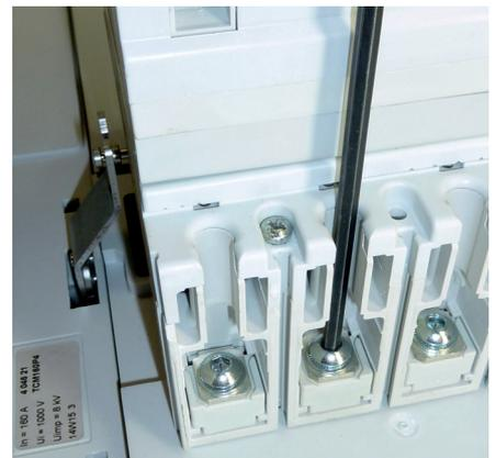
Tighten the upstream and downstream electrical connections with the eight (or six) screws provided with the base (tightening torque: 7N·m -> DPX<sup>3</sup> 160; 10N·m -> DPX<sup>3</sup> 250; 24N·m -> DPX<sup>3</sup> 630).
