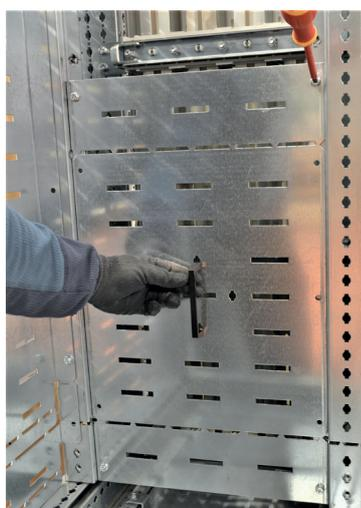
The cover plates are manipulated with a removable handle supplied in the kit. They are screwed onto the side partitions.
