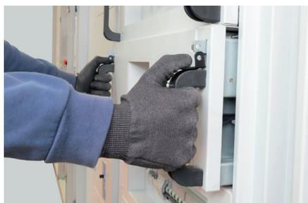
To fully insert the tray, apply pressure to both locking levers and push in the tray.
