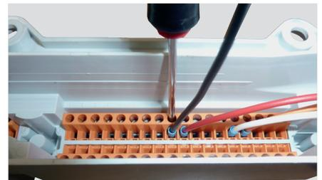
Connect the outgoing lines for the auxiliary circuits equipped with Starfix ferrules, using the same wiring diagram as for the movable part.
