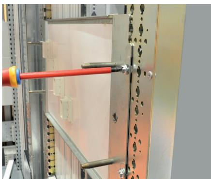
Place the fixed part in position and fix it on the IS chassis functional uprights.
