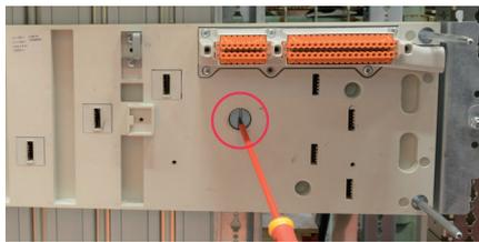
This ¼ turn lock, in the middle of the fixed part, prevents the base being removed while the circuit breaker is in place.
