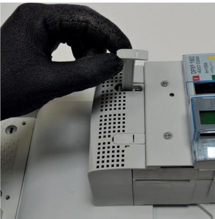
Lock the terminal shield by inserting the two sealed locking caps.
