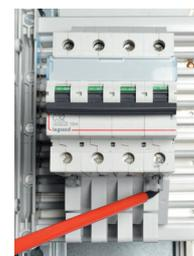
The circuit breaker is correctly installed once it is locked onto the rail.
