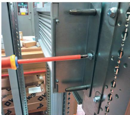
Complete installation by securing the movable part to the fixed part with the two screws supplied.
