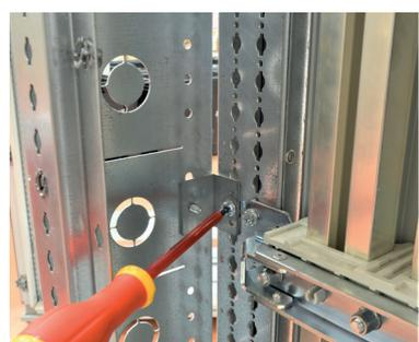
Fix the side partitions on the four previously installed lugs.
