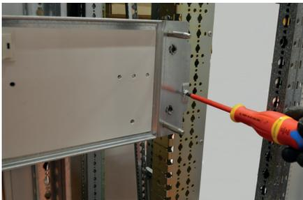
Then secure the fixed part using the screws supplied with the row distribution block.
