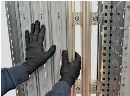
The insulating strips are first inserted in the lug support guides. They are then clipped onto the busbars starting at the bottom, exerting pressure on the sides.
