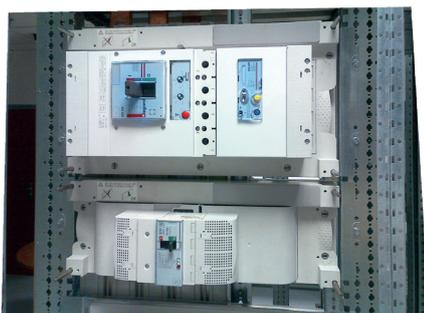
DPX and DPX<sup>3</sup> circuit breakers are mounted horizontally on the bases.
