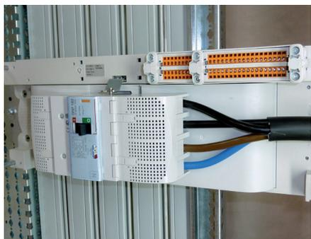
Install the downstream terminal shield, and insert both locking caps (in this photo, the circuit breaker has a rotary handle).
