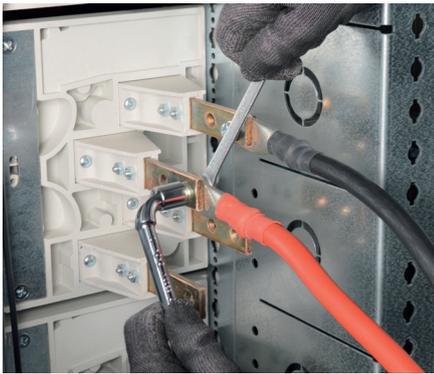
The IS 233 bases are connected downstream using bar ends with two drill holes for M8 screws, enabling connection via bars or lugs.
