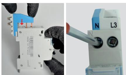
Install the module in the same way as on the automatic terminals so that the prongs of the connection module fit into the circuit breaker terminals and then tighten to torque (1.6 to 2 Nm).
