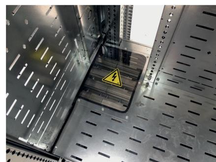
Example of horizontal busbar at the bottom of the enclosure with access cover created by the panel builder for checking the fish-plating.
