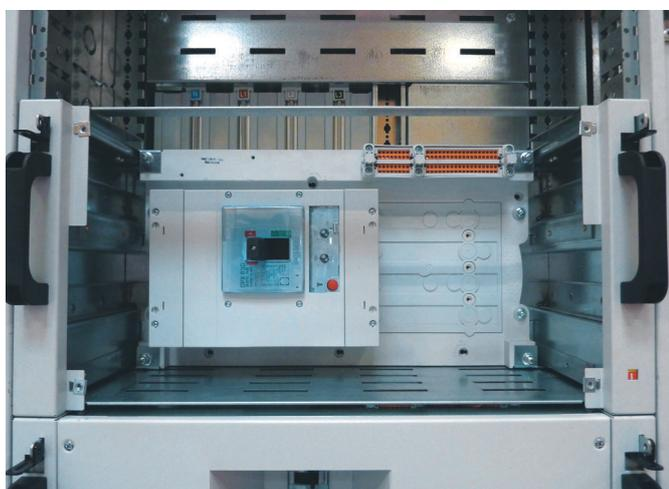
The drawer (movable part) is inserted in the same way as the one on the DPX<sup>3</sup> 250 (see page 47), by exerting pressure on both locking levers.
