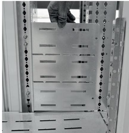
By default, spare compartments must be fitted with dividers (Cat.No 4 046 89) which can achieve form 3b, the minimum level required for IS 233.
