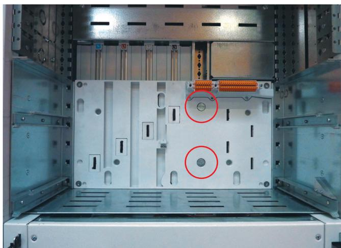
The base (fixed part) is inserted in the enclosure in the same way as the one on the DPX<sup>3</sup> 250 (see page 46), except that it is locked with two ¼ turn screws.
