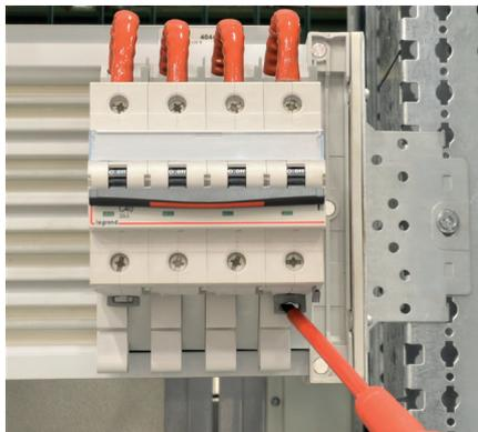
Complete installation by locking the circuit breaker clips.
