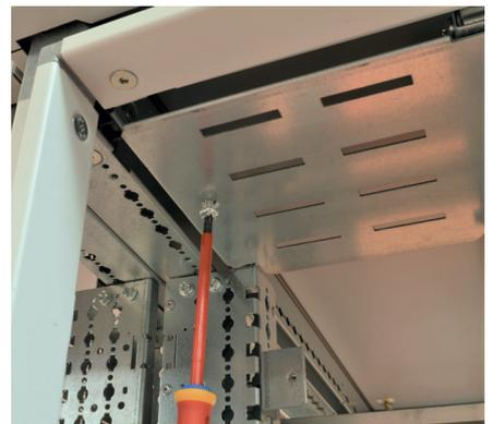
The top and bottom dividers are screwed onto brackets (two at the top and two at the bottom). These are fixed on the structural uprights 100 mm from the front of the enclosure.
