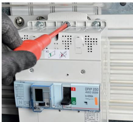
Complete installation of the DPX<sup>3</sup> by locking the 1/4 turn screws above and below the circuit breaker.
