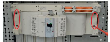
The movable part is locked onto the fixed part using the ¼ turn screws (two on each side).
