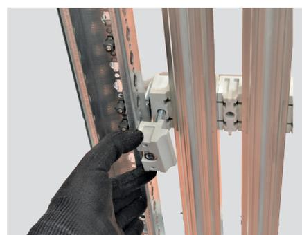
The busbars are engaged in the isolating supports. Flanges screwed into the supports hold the busbars in position.
