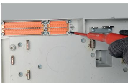
For the movable part, the female part of the connection module is fixed at the rear with six small screws (tightening torque 2.5 N·m).
