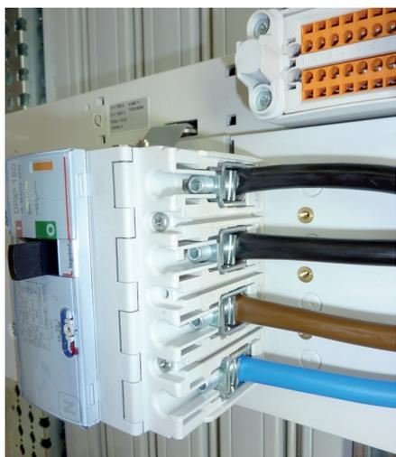
Connect the cables in the circuit breaker downstream cage terminals (tightening torque 8 N·m).
