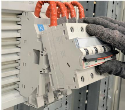
Engage the MCB in the same way as onto a standard DIN rail.
