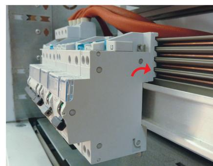
Position the circuit breaker on the rail by first pushing in the bottom of the appliance, then exerting pressure on the top to push the circuit breaker into position. The product is then automatically connected to the distribution block.
