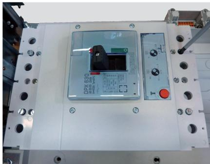
Fix it using the four screws supplied with the circuit breaker (tightening torque: 1 N·m).
